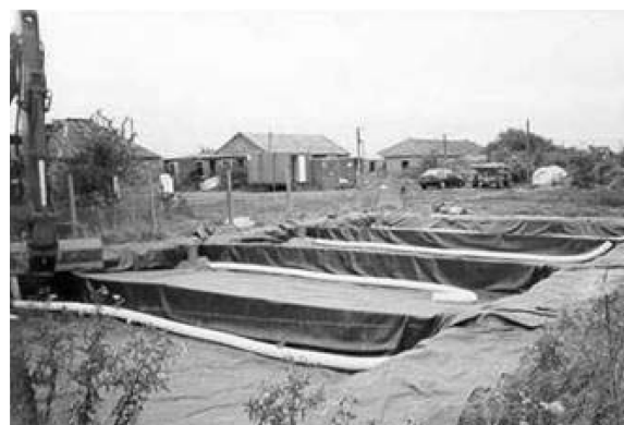
Fig. 1 Construction of four pilot-scale cells in the site. Cell 1: untreated soil; Cell 2: EnvirOceM soil; Cell 3: OPC soil; Cell 4: ACT soil.
